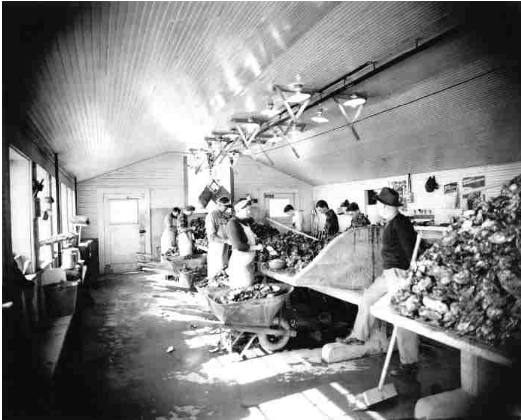
Figure 27 Rock Point Grading Room (Steele).
