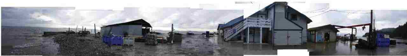
Figure 41 Existing site conditions viewing west. from left to right: storage, existing retail and dock (Author).
